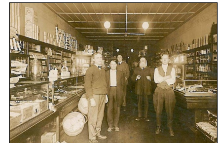
INTERIOR OF STEPLETON GENERAL STORE
