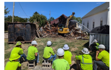
Apollo students working on the demolition of the house adjacent to the museum.
